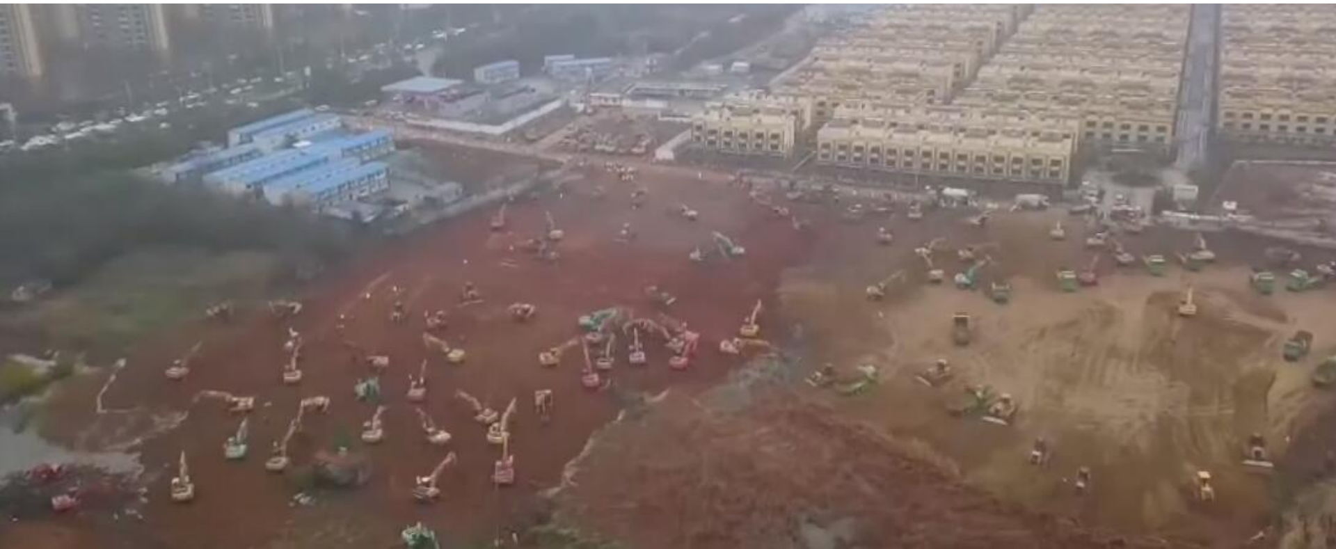
Construction site of Huoshenshan Hospital as of 1/24
